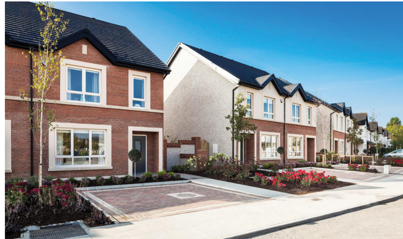
Figure 65. Sample image of similar building finishes. Comparable size development delivered by Liscove Limited .
