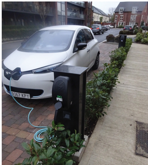
Figure 62. Sample image of vehicular e-charging points .
